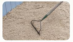
**Hand Rakes** for leveling ThorTurf around edges and walls.
